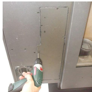
Fig. 42 - Inspection panel removing
