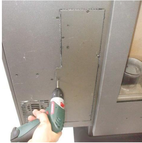
Fig. 43 - Heat protection panel removing
