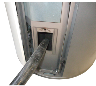
Fig. 53 - Fume passages cleaning
