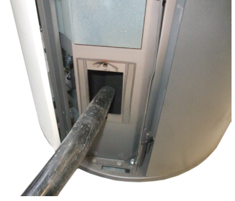
Fig. 62 - Fume passages cleaning
