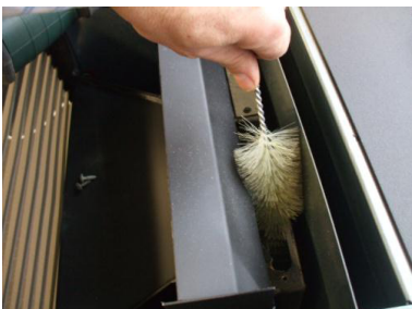
Fig. 45 - Fume passages cleaning
