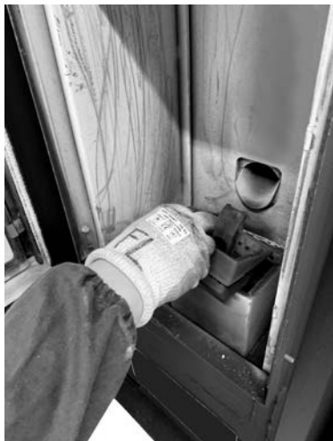
Fig. 27 - Burning pot extraction
