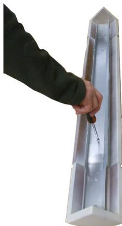
**Fig. 26 - Tighten the profile to the tiles**
