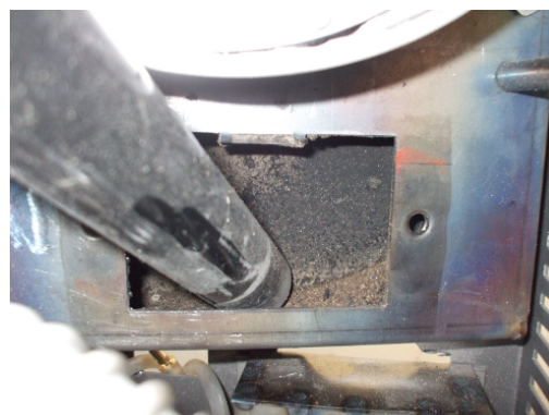
Fig. 35 - Fume chamber cleaning
