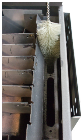
Fig. 43 - Fume passages cleaning
