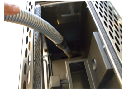
Fig. 23 - Combustion chamber cleaning
