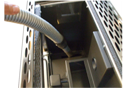
Fig. 22 - Combustion chamber cleaning
