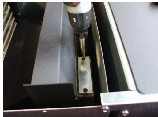
Fig. 39 - Lids removal
