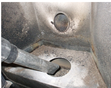
Fig. 28 - Burning pot box cleaning
