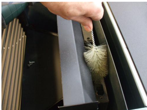
Fig. 40 - Fume passages cleaning
