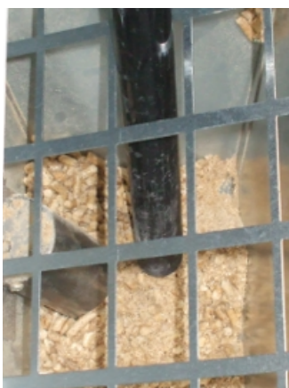
Fig. 31 - Hopper and auger cleaning
